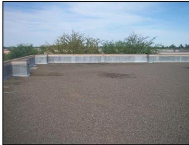
that many of the roofs had originally been installed with less than code required slope. Some areas were even found to slope away from drains and evidence of ponding was observed. The jurisdiction did not require issuance of permits for building re-roofing.
